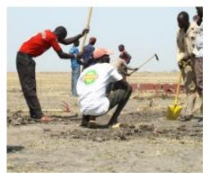
or foreseen. The helical pier foundation was not successfully installed in the first phase because of issues with our installation tool. We plan on addressing this with the manufacturing company and utilizing the piers for the flooring system. We relied on our Plan B for the foundation and hand dug 46 holes for a concrete steel combination footing.
